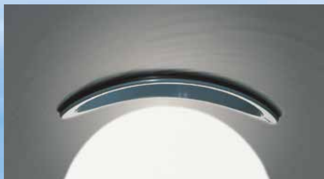
Internal view of a CONNEX PVC-U DN/OD 400 sewer pipe with correctly fitted CONNEX-Junction (internal view)
