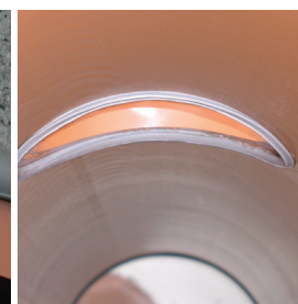
Correct installation of the junction.
