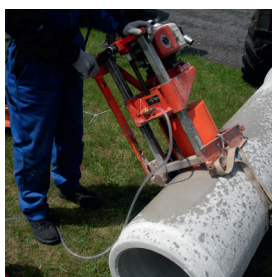
Correct Coredrilling
